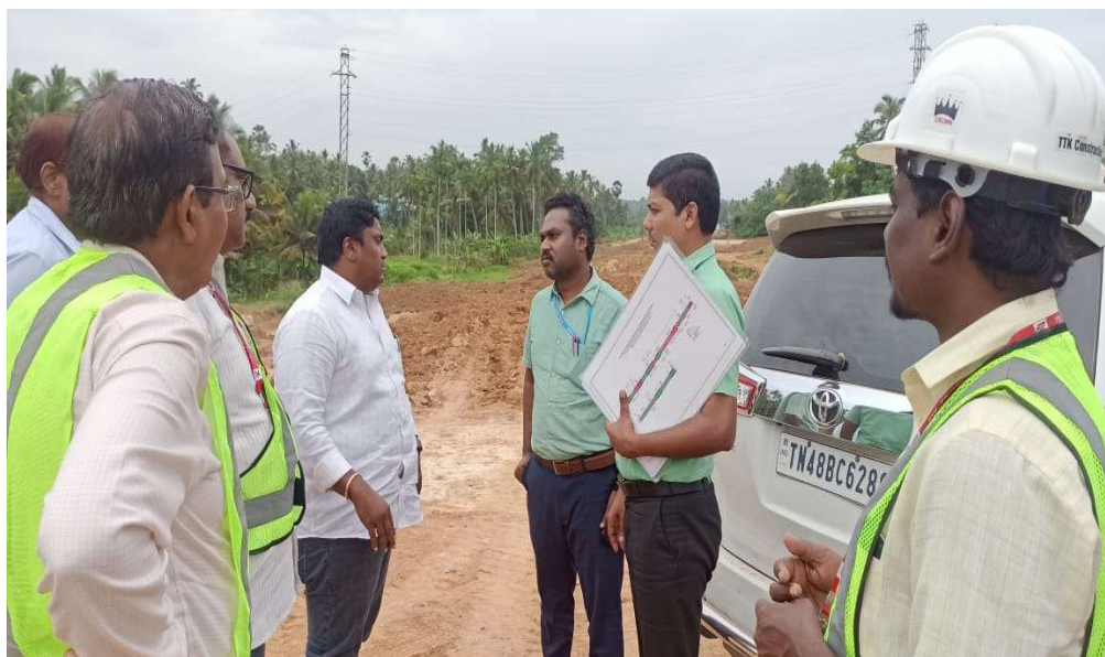
SITE VISIT CONDUCTED BY THE REGIONAL OFFICER, NHAI, MADURAI IN PROJECT OF FOUR LANING OF LEFT-OVER WORKS INCLUDING ADDITIONAL STRUCTURES IN KERALA / TAMIL NADU BORDER - KANYAKUMARI (NH 47) AT NAGERCOIL
