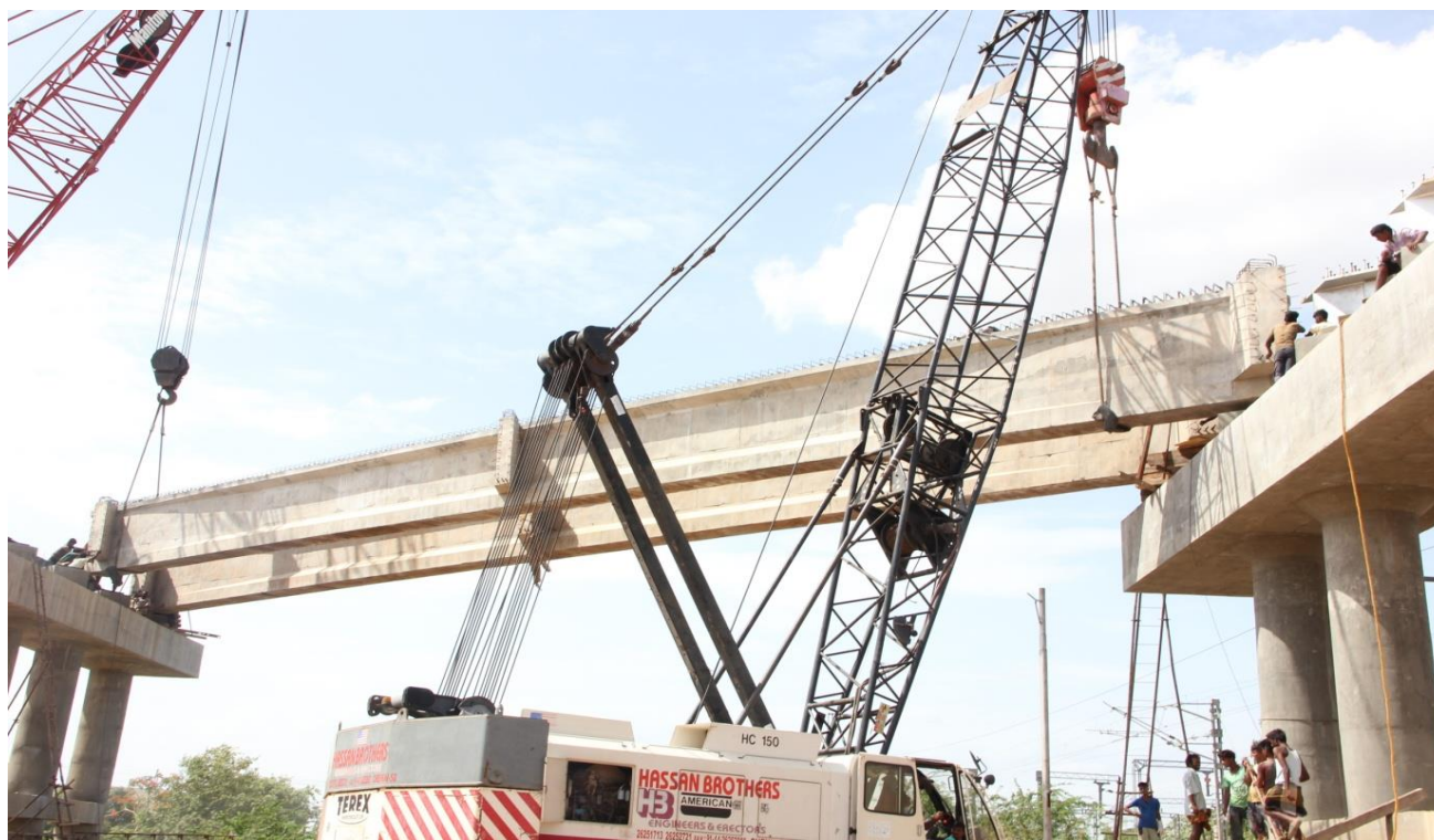
Road Over Bridge in Lieu of Exg. LC No. 201 at KM: 271/0-1 between Ariyalur and Sillakkudi Stations. Composite Girder - 1 X 44.0m and PSC I Girder - 2 X 31.0m
