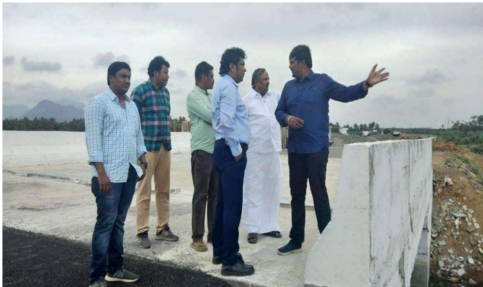
INSPECTION OF THE PROJECT DIRECTOR, NHAI, NAGERCOIL IN NARIKULAM TANK CONSTRUCTION AT MADURAI - KANYAKUMARI SECTION OF NH44 (OLD NH-7) IN THE STATE OF TAMIL NADU
