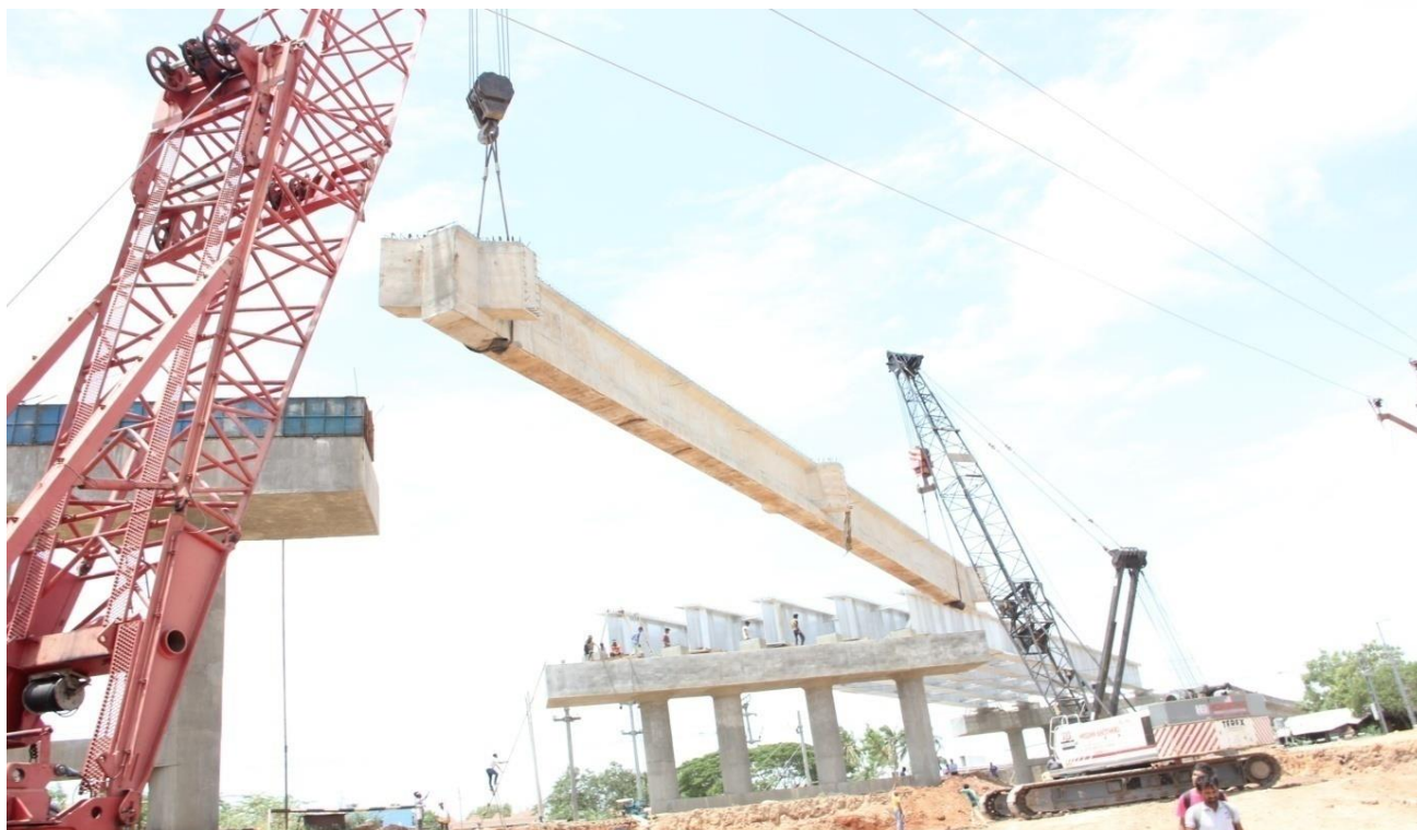
Road Over Bridge in Lieu of Exg. LC No. 201 at KM: 271/0-1 between Ariyalur and Sillakkudi Stations. Composite Girder - 1 X 44.0m and PSC I Girder - 2 X 31.0m
