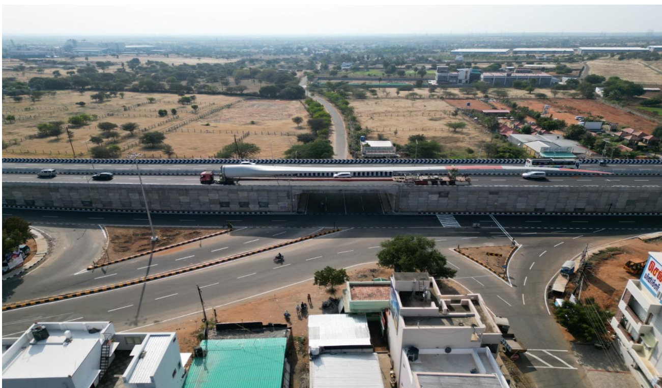
VUP at Karur - Dindigul Road NH-7
