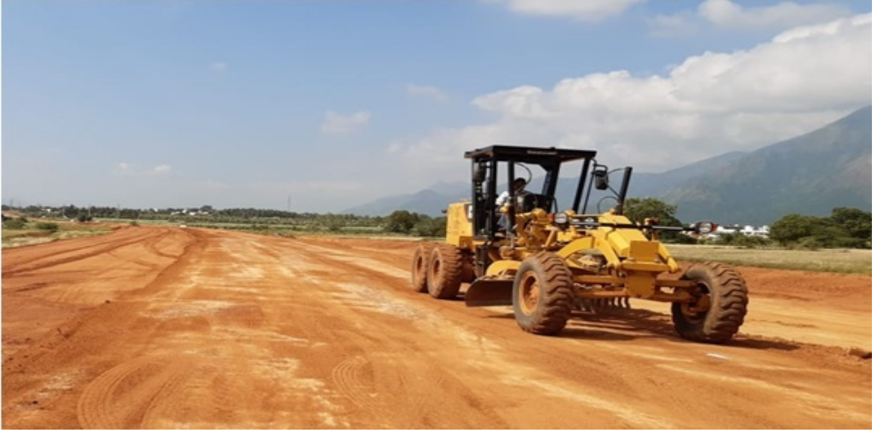
Embankment Grading
